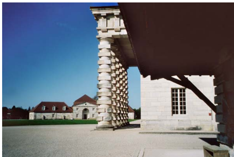
Ill. 7, The diagonal strut on a berne corner
